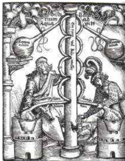
Below: the title page of a work written by Hieronymus Brunschwig hi 1507 on the art of distillation. Although European alchemists spent much time and ingenuity on the arrangement of their stills, the art was developed, if not invented, by the Arabs, and it became an enormously important process.
