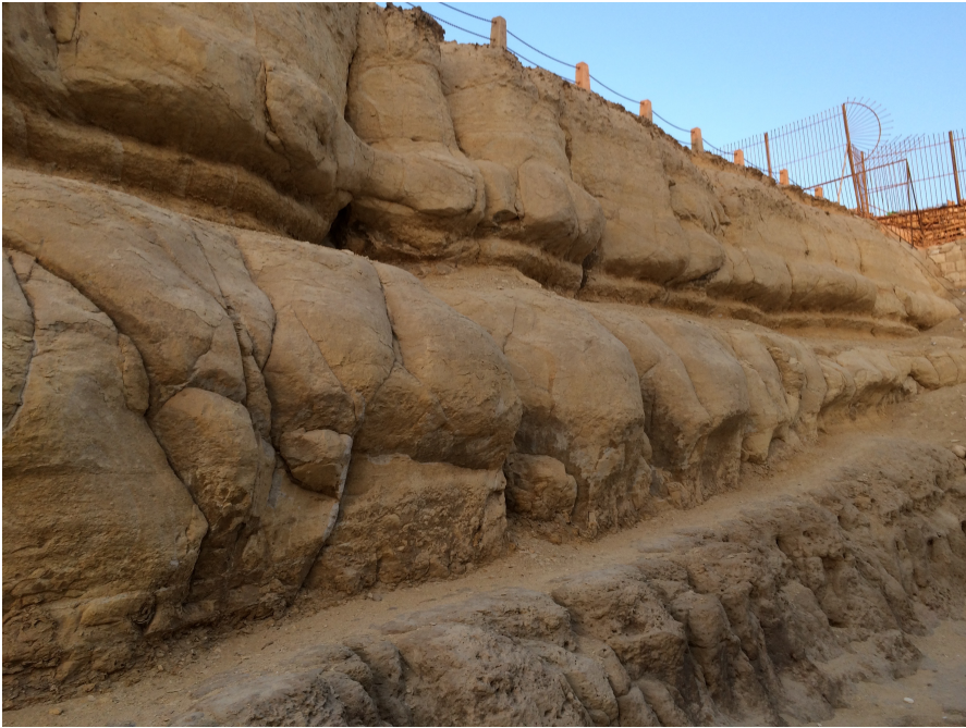
Illustration 4: Rain induced weathering on the southern wall of the Sphinx Enclosure. TG
