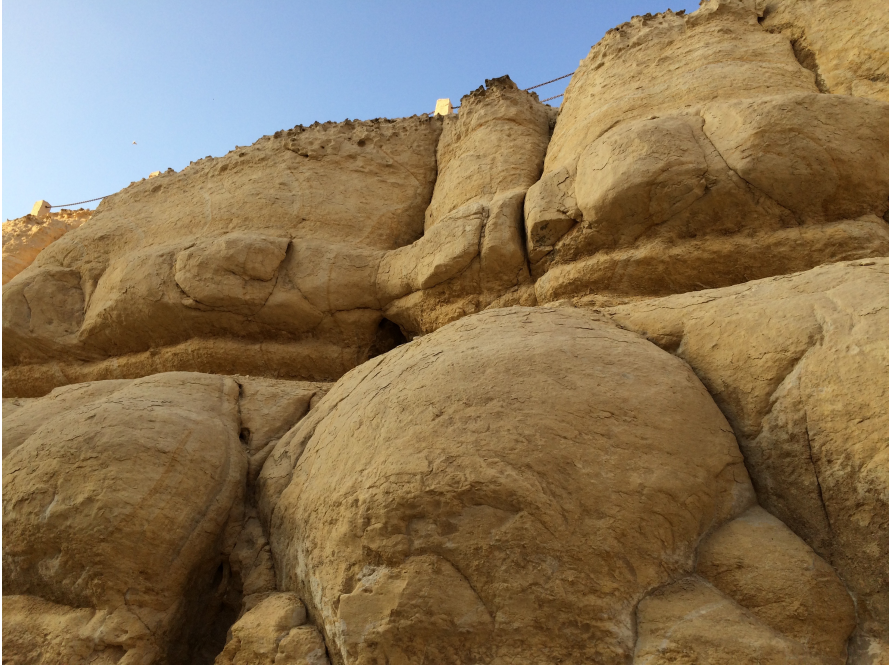
Illustration 3: 'Textbook example' of precipitation induced erosion on the southern enclosure wall of the Sphinx courtyard. TG
