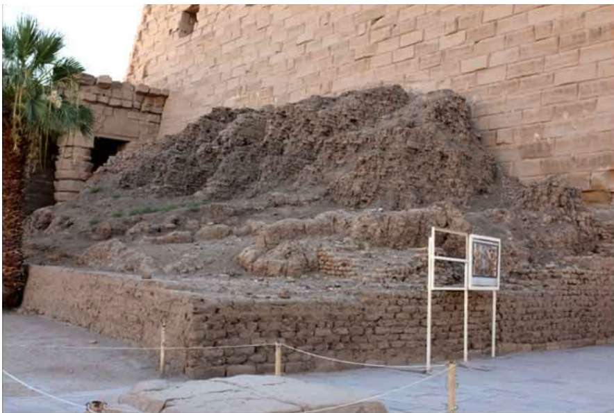
Illustration 2: Interior view of the wall near the entrance of ram-headed sphinxes at the Karnak Temple Complex. Dried mud bricks are piled against the wall.
